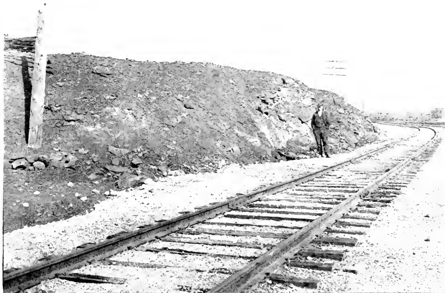
The photograph illustrates how the building of the Canadian Pacific Railway was the means of discovering a great nickel-copper mine; namely, the Murray. The railway cut intersects the ore body, the latter being shown to the left of the track beside the man. Photograph taken Sept. 2nd, 1916.
